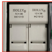
Fuse protection Positive and negative poles protected against overcurrents by gPV fuses.
